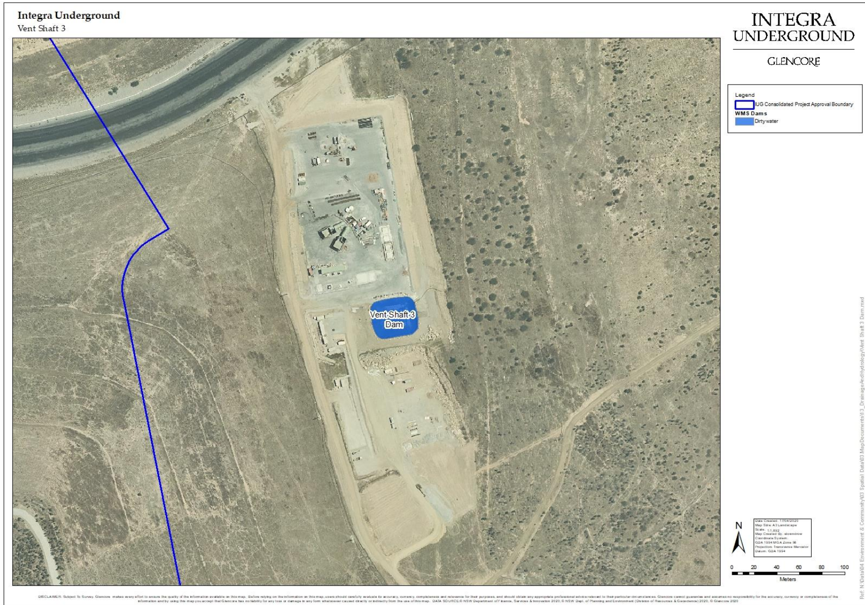
Figure 4 – Vent Shaft 3 Dam
