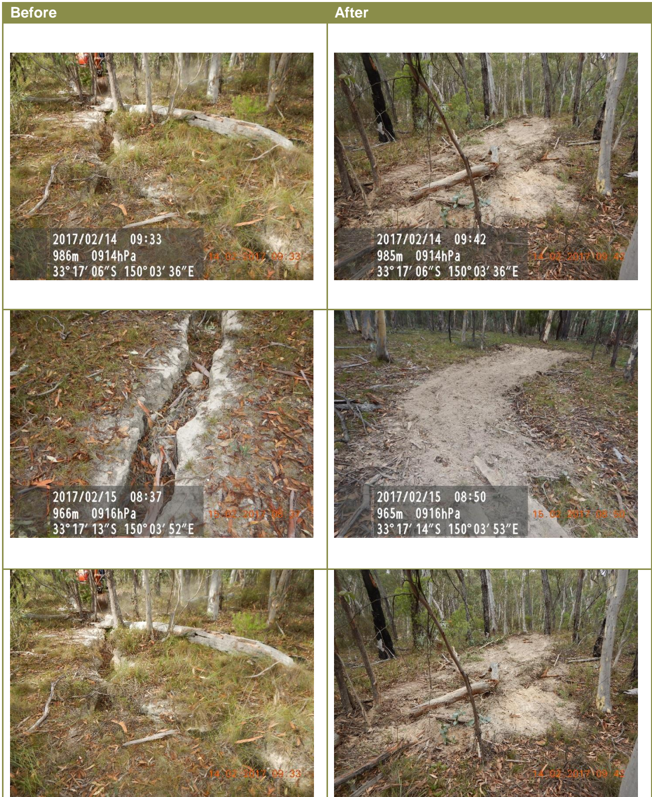
Plate 1: Before and after photos of shallow cover subsidence repairs in February 2017.
