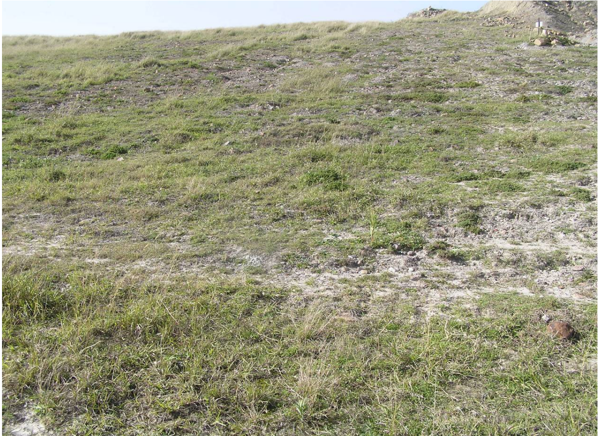
Plate 11. Railway block. Bare failed areas need ripping and reseeded. Entire domain needs fertilising to improve health of pasture sward. Spray Galenia patches.
