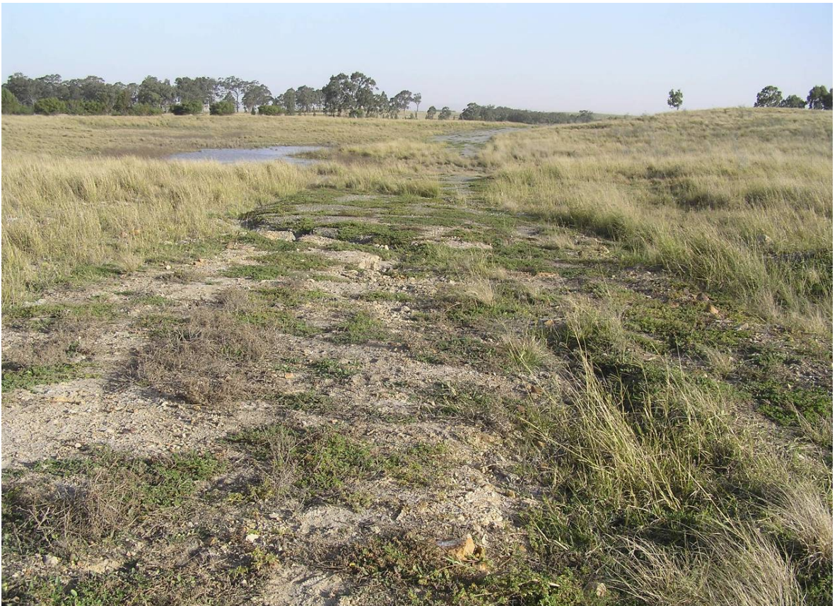
Plate 26. Mountain Block. Decompact and seed old haul road. Locate and infill sink holes (mostly around dam) in this vicinity.
