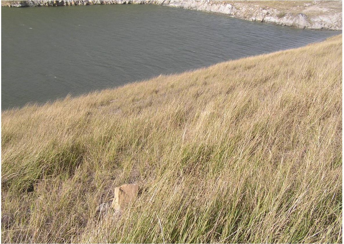
Plate 19. Antienne East. Example of good pasture cover and slope stabilization on difficult area around dam. A good pasture cover reduces potential for weed invasion (particularly Pampas grass in these areas).
