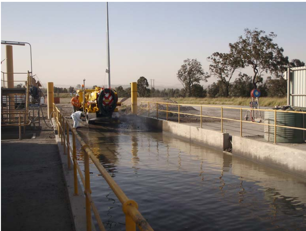
Plate 2 Liddell new light vehicle wash down bay
