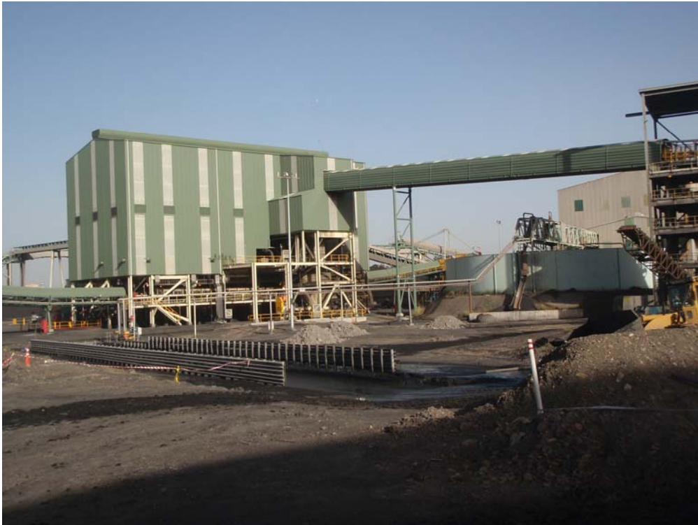
Plate 9 New Liddell CHPP
