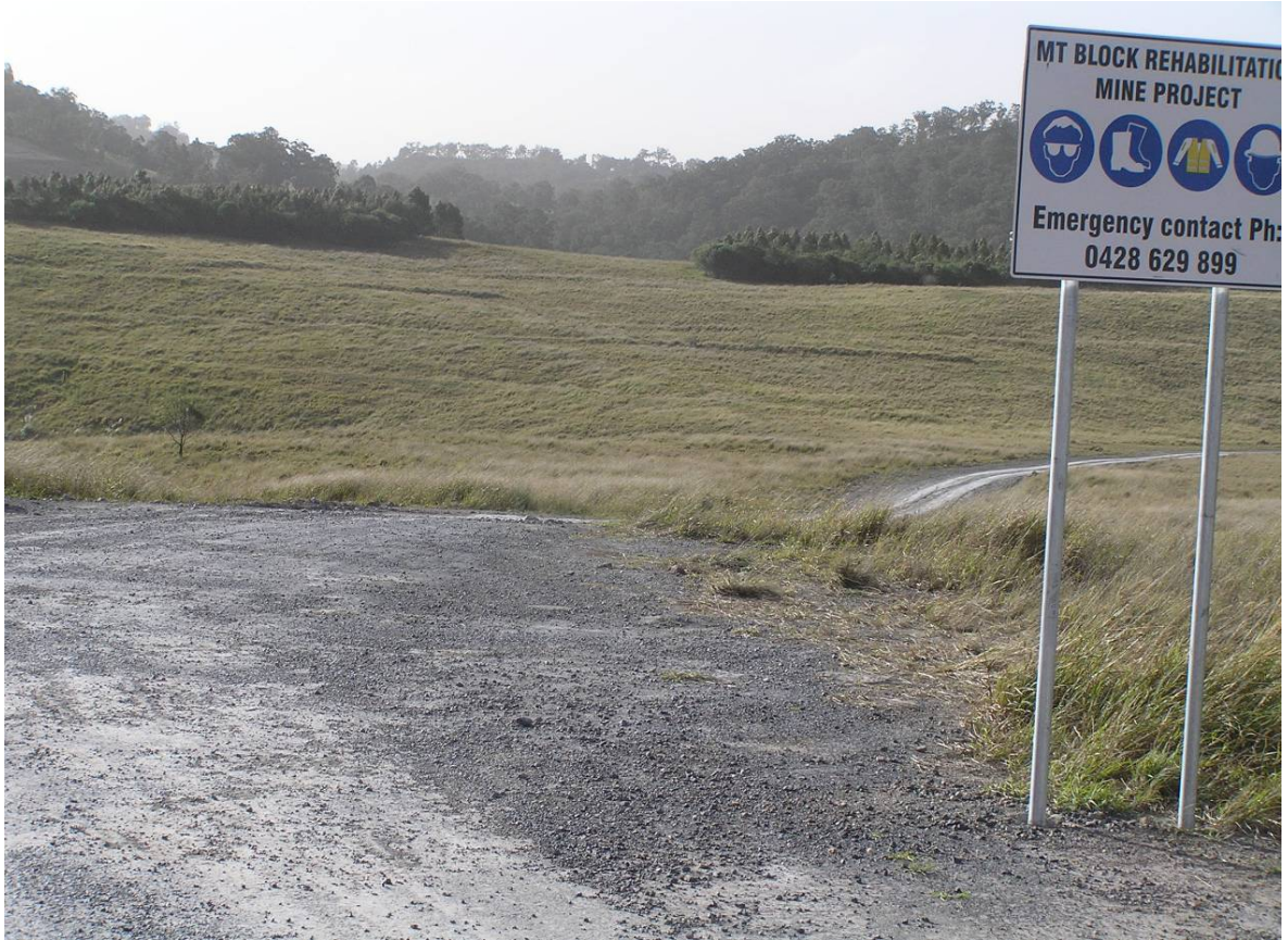
Plate 23. Mountain Block. Pasture and tree areas in this domain would benefit from weed control and maintenance fertilizer
