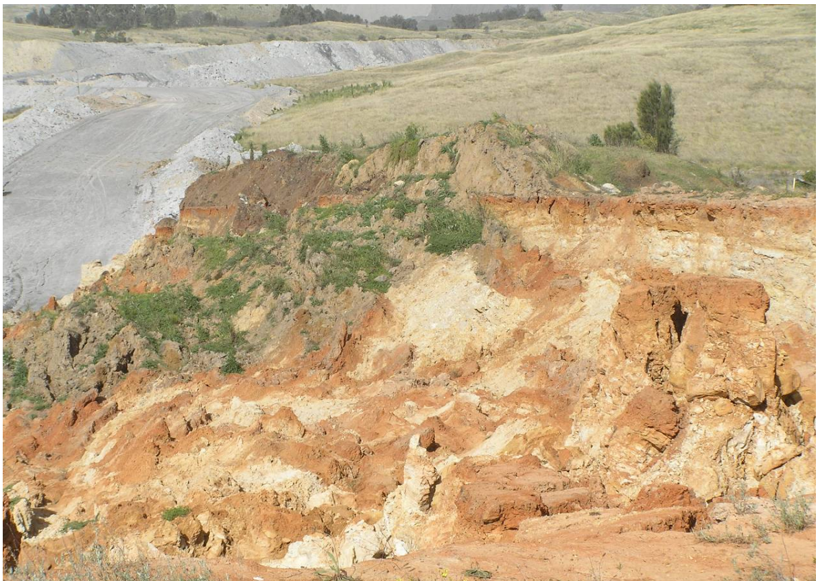
Plate 12. Reservoir Block. Topsoil stockpile largely lost into pit. Recover remnant soil and improve topsoil recovery and management generally across mine.
