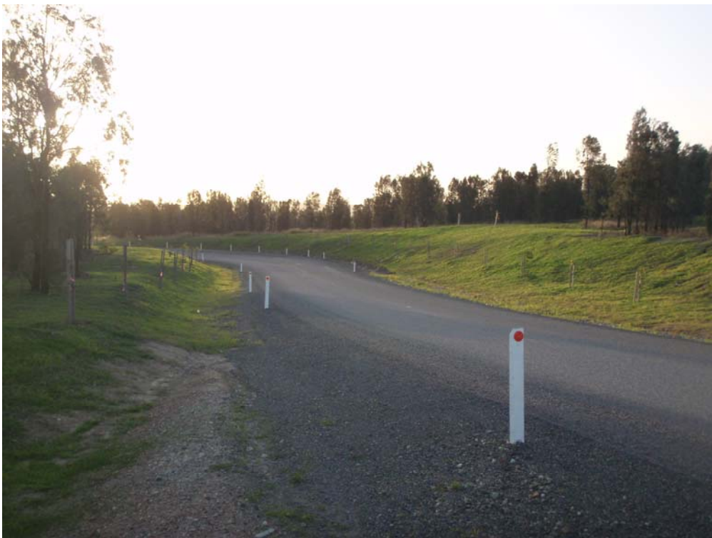
Plate 6 Liddell Access Road
