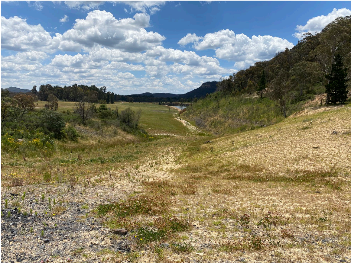
Photo 10 – Good rehabilitation along steeper sections of site.
