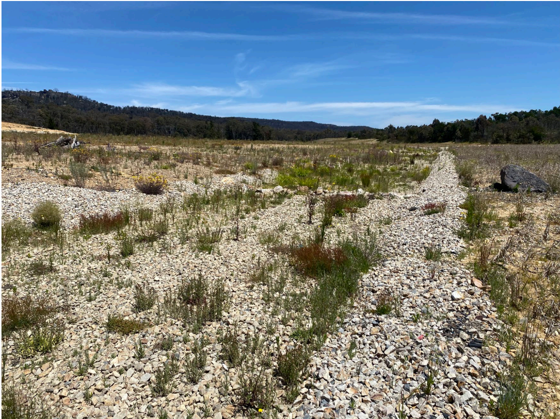
Photo 3 – Good use of recycled railway ballast used in engineered drains.
