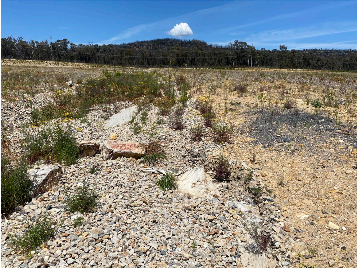
Photo 5 – Minor erosion along drains exposing geo-fabrics.
