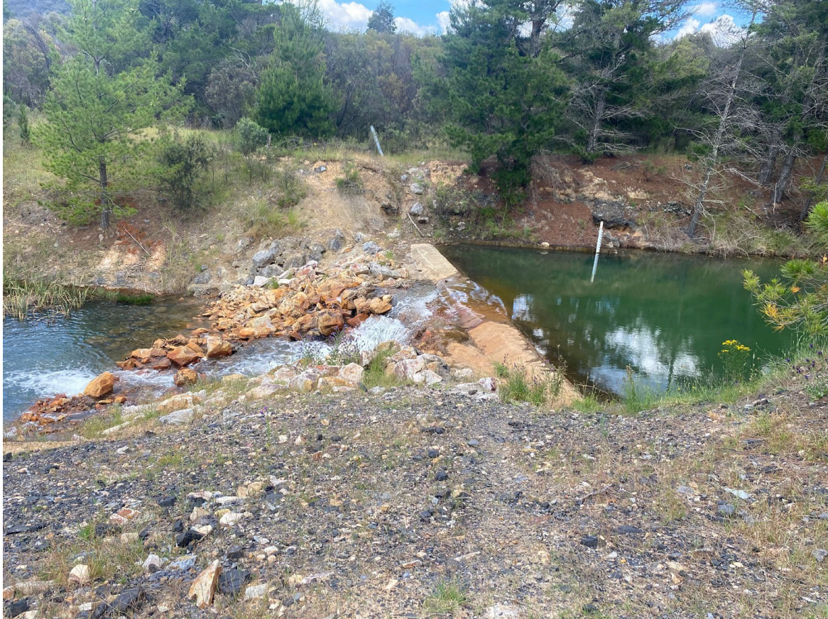
Photo 11 – Overshot dam spillway.
