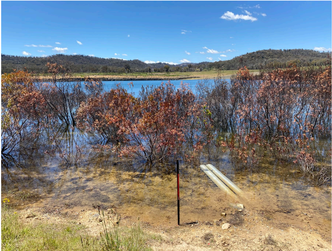
Photo 7 – Drainage pipes from final void to control water height.
