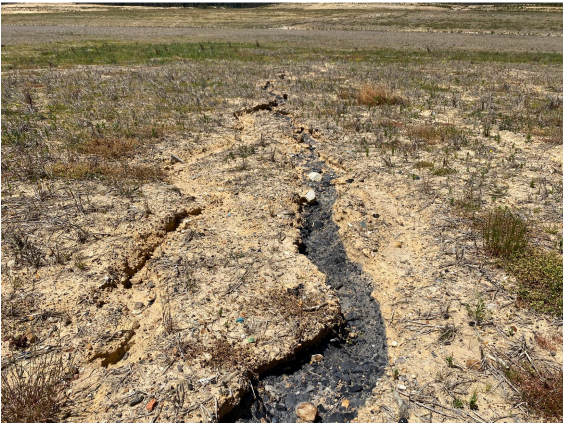
Photo 4 – Areas of erosion that require remediation works. Note the site had approval under the Detailed MOP for a low capping cover.
