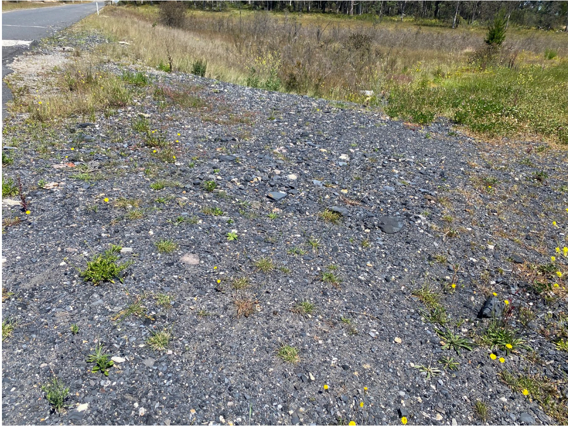
Photo 9 – Minor rehabilitation still required in small areas of the site.
