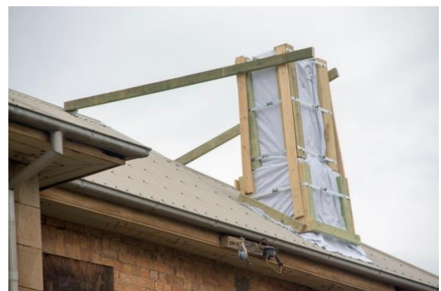
Figure 13 Annex chimney stabilisation framing
