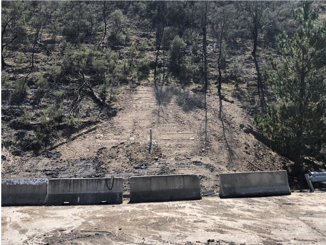
Plate 3 Example of repaired adit entry site (Source: Minesoils, 2020)
