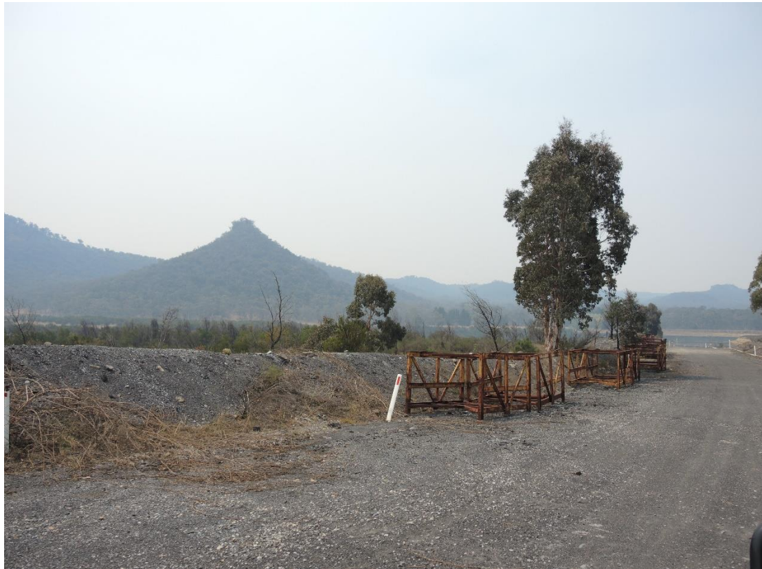
Plate 16 Scrap steel located near Dirty Water Dam requiring re-cycling
