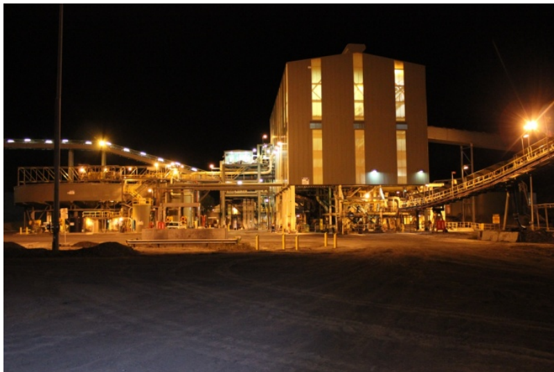
Internal site 3 (night) facing south towards CHPP
