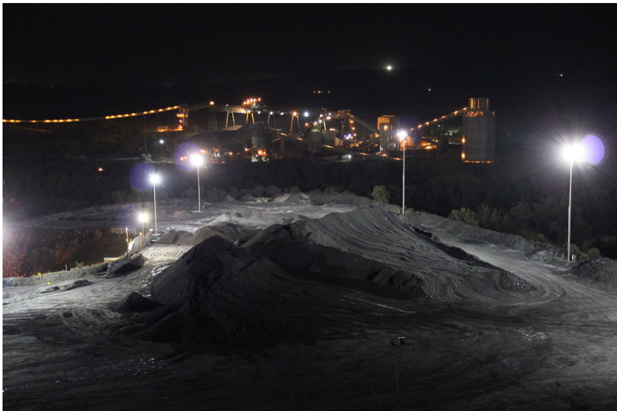
Photograph 3.1 Large free-standing lighting structures to product stockpiles
