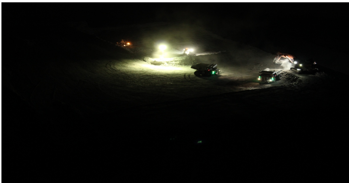
Photograph 3.4 Lighting on excavators and haul trucks reduce need for additional lighting
