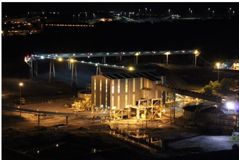
Internal site 2 (night) facing south-east over CHPP
