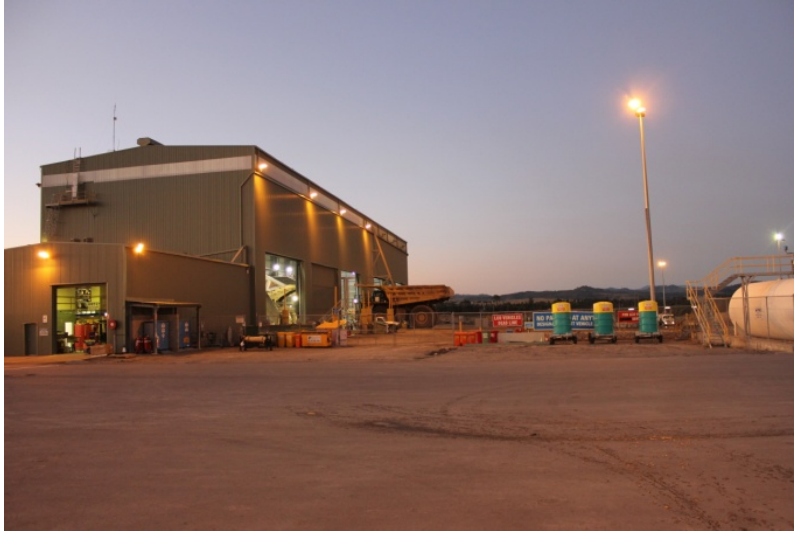
Maintenance area and shed (day)
