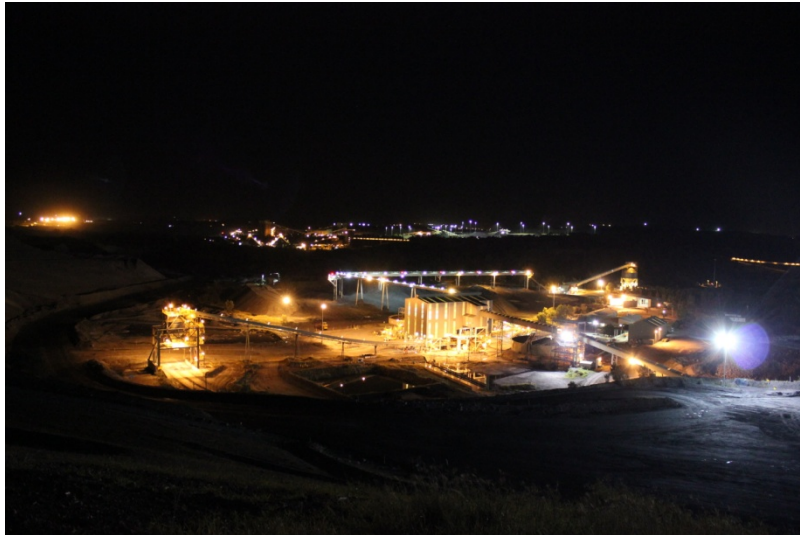
Internal site 2 (night) facing south-east over CHPP
