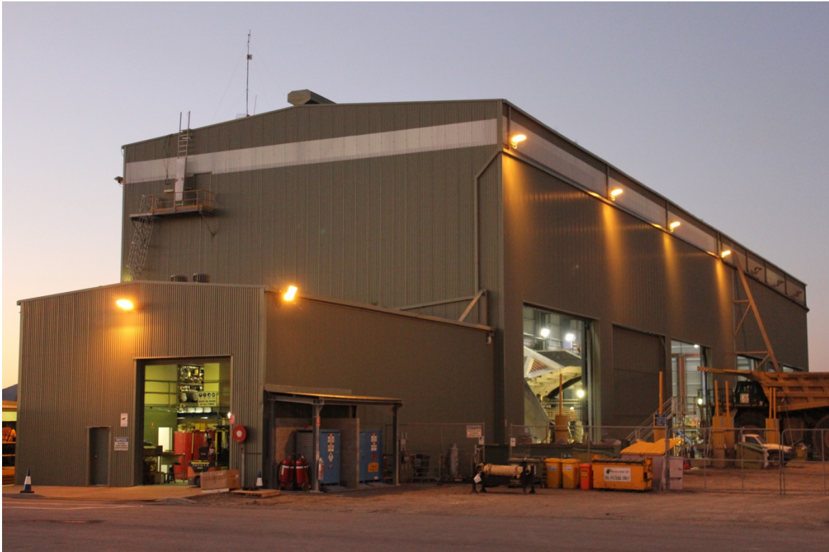
Photograph 3.2 Fixed lighting structures
