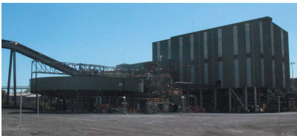
Liddell Coal's new Coal Handling and Preparation Plant
