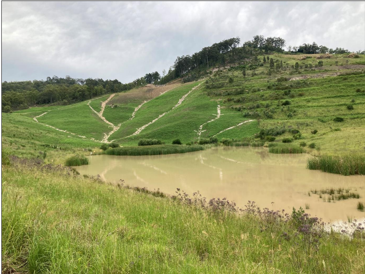
Figure 9-8 – Mountain Block Rehabilitation after completion of earthworks and seeding (February 2021)
