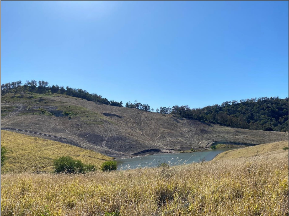
Figure 9-7 – Mountain Block during major earthworks (August 2020)
