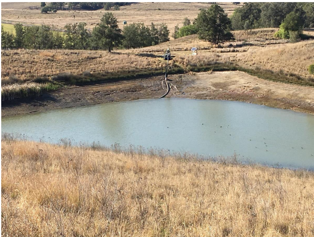
Figure 5 – From the top, photos of Dam 6 facing ENE and SE respectively.
