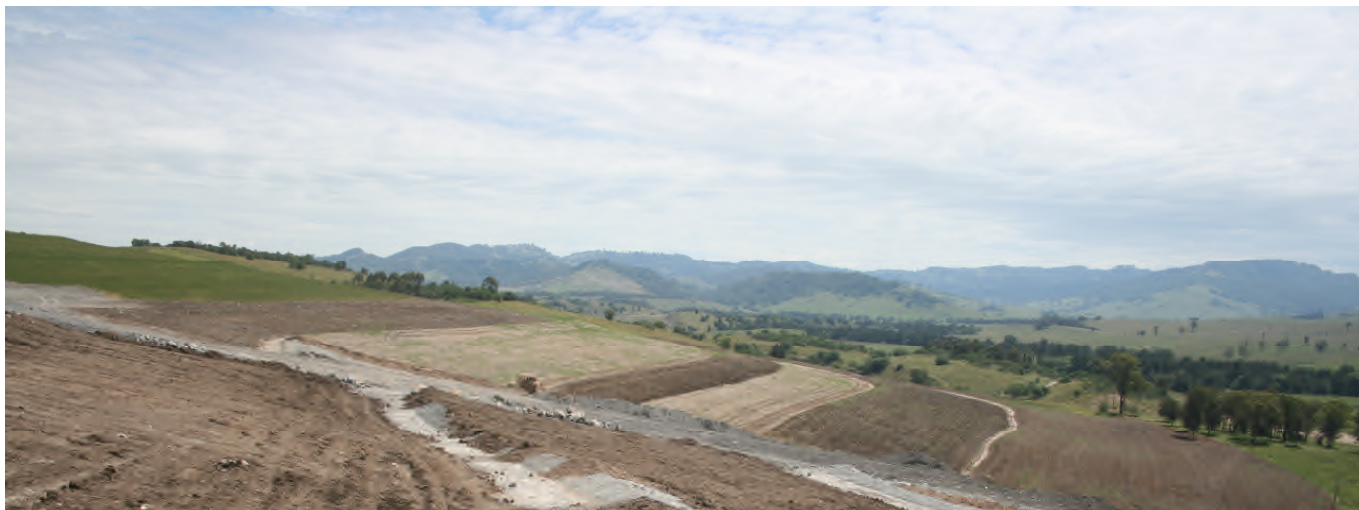
Plate 13: Cross tilled rehabilitation at Premier Dump
