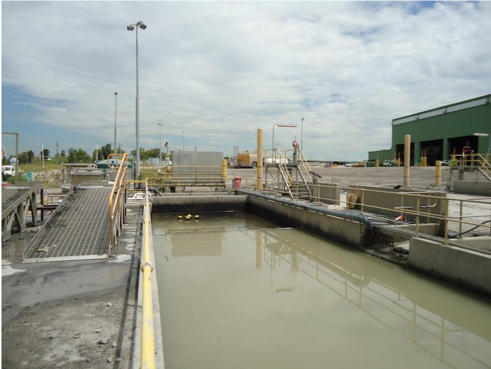
Plate 5 Vehicle Wash Down Sumps
