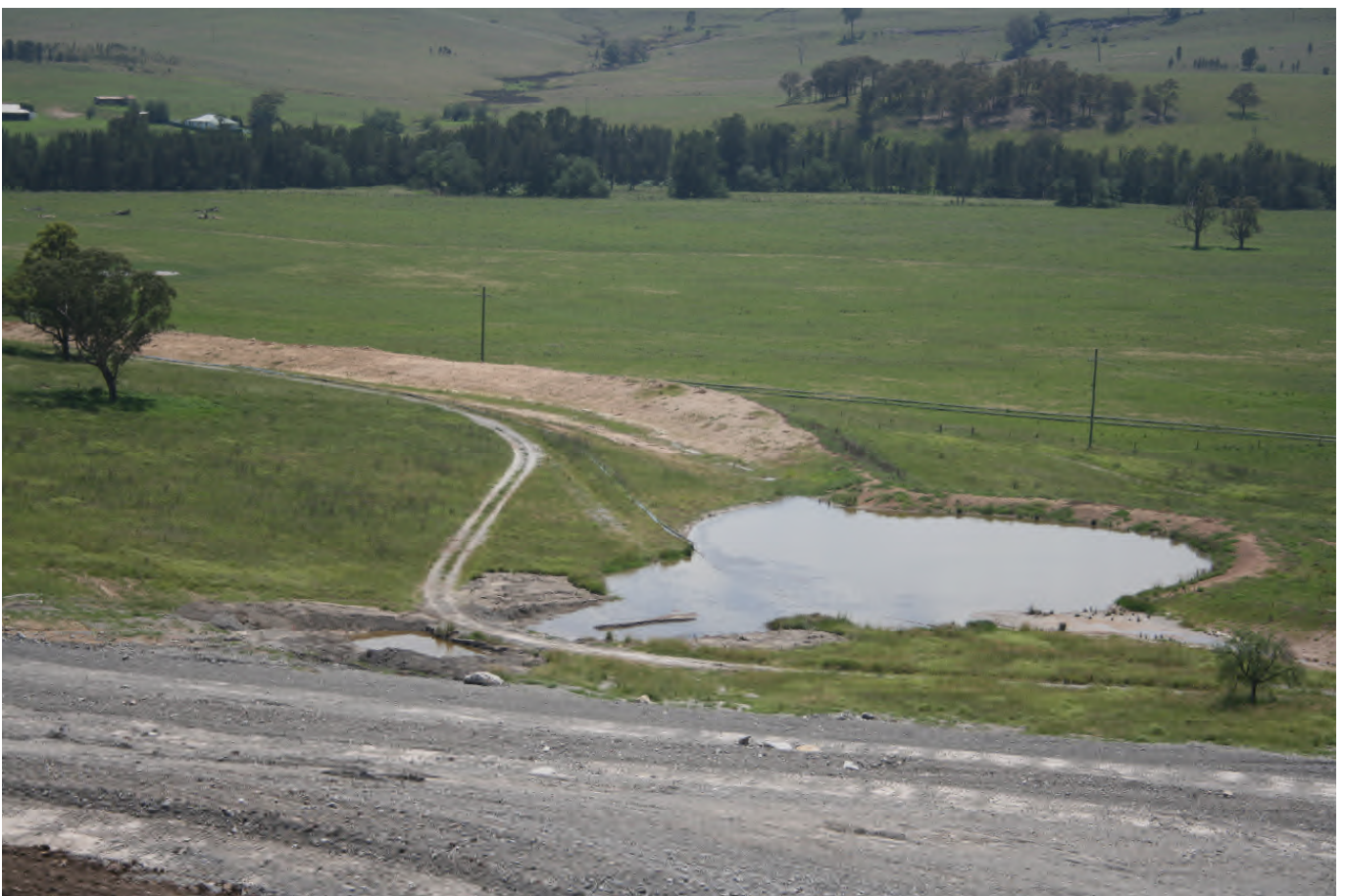
Plate 12: Premier Dump sediment catch drain
