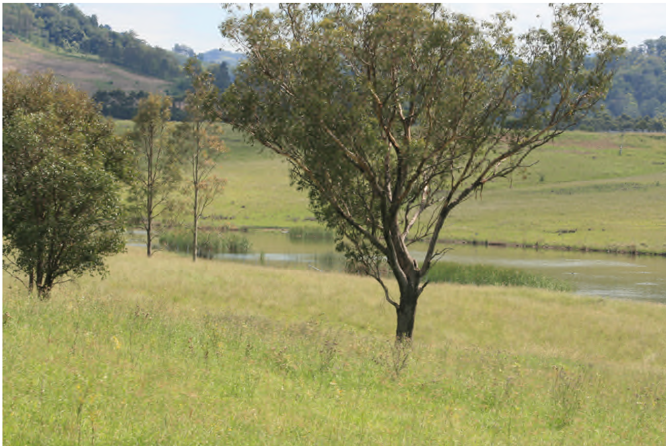
Plate 5: Dam 3 banks less than 10 degrees
