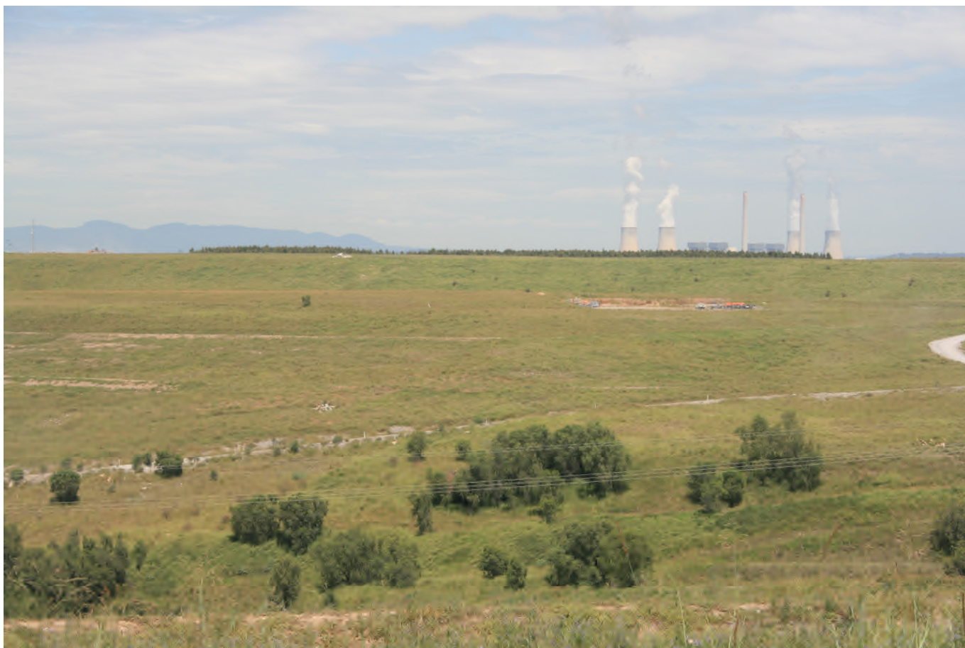
Plate 14: Level surface of RL 195 Dump
