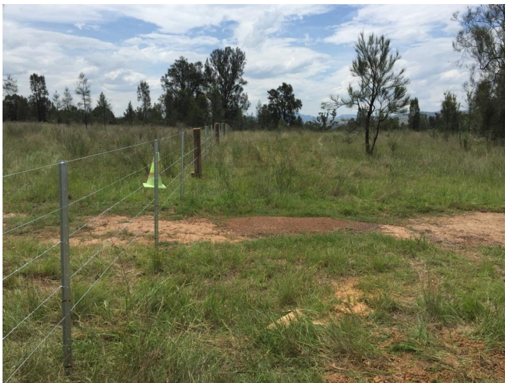
Plate 16 Bowmans Creek SAL Fencing (underway at the time of audit)
