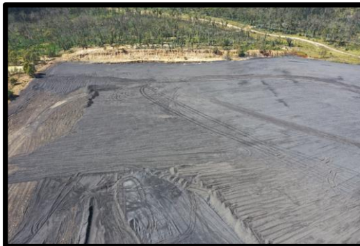
Leachate Dam – February 2021
