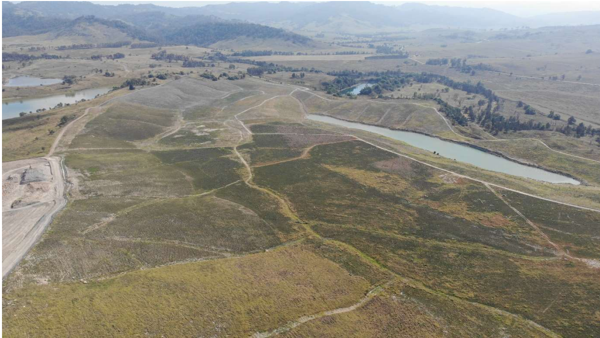
Figure 8-3 - Completed Antiene and Dam 4 Rehabilitation
