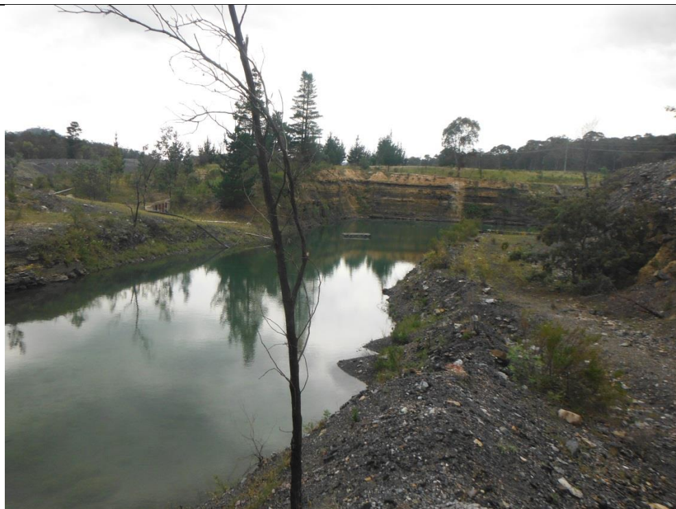
Photo 6 – Dirty Water Dam
