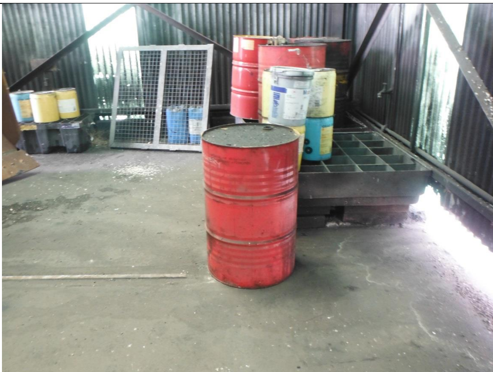
Photo 14 –Chemical Container not stored within a bund
