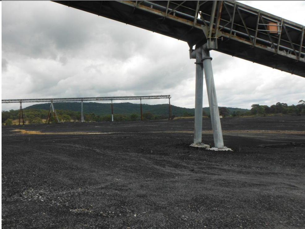
Photo 5 – CHPP and Stockpile Area
