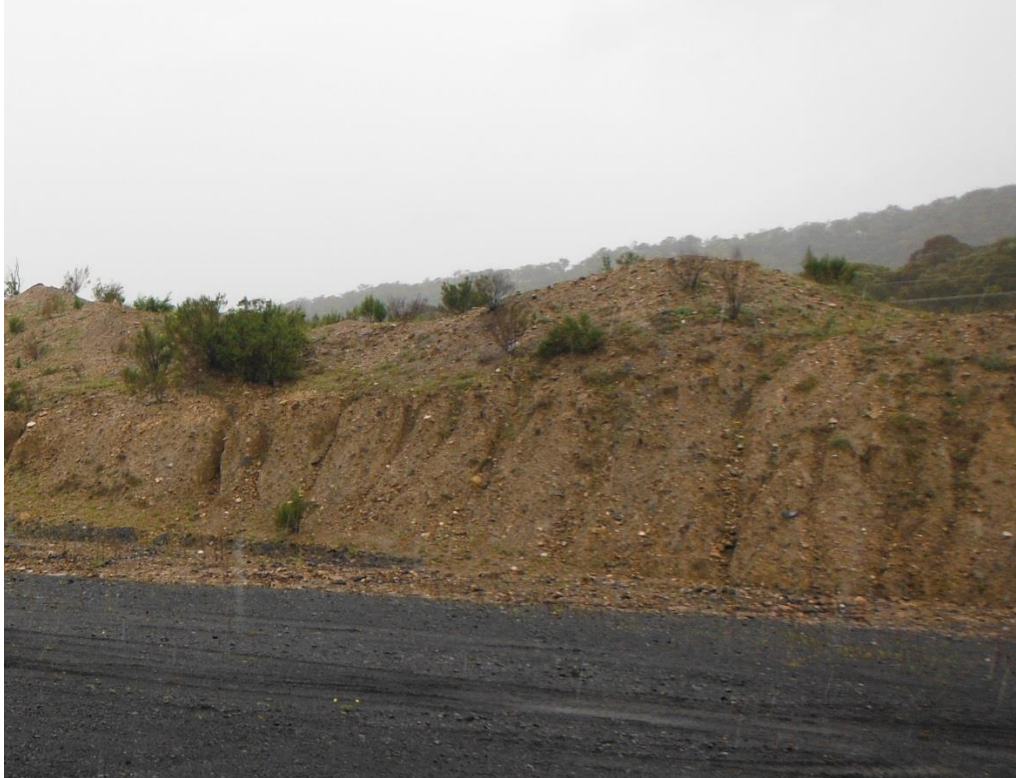
Photo 11 – Soil stockpiles should be seeded to reduce erosion potential.
