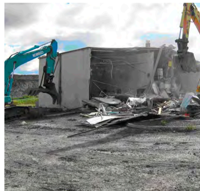
Demolition of the mining contractor open cut bathhouse and crib facilities.
