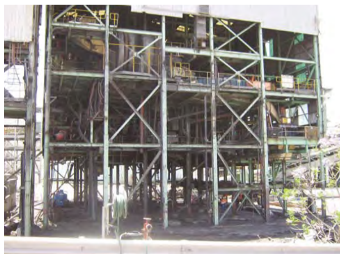
Deconstruction of the old Coal Preparation Plant.
