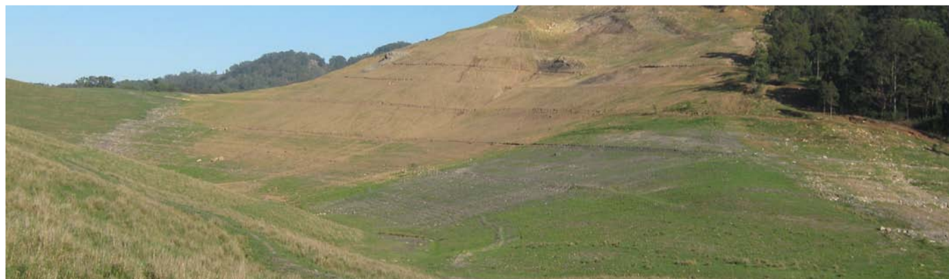
Rehabilitation work at Mountain Block.
