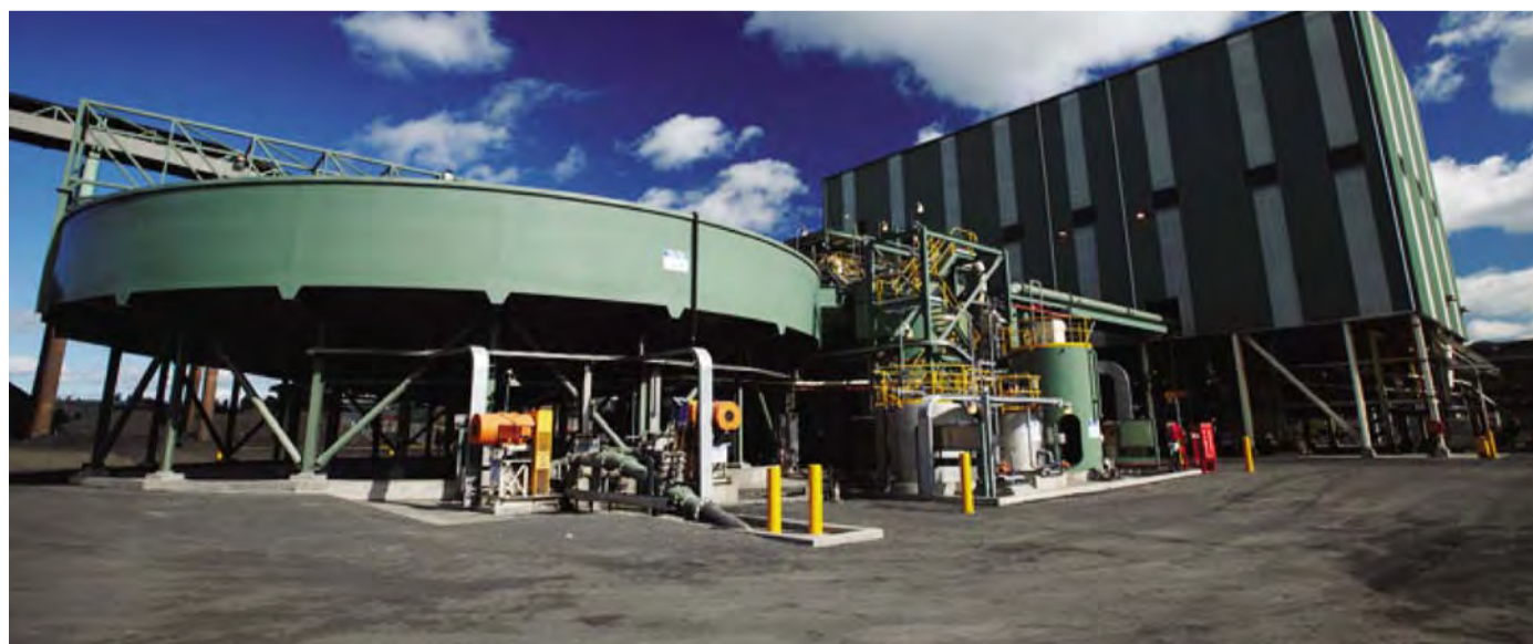
New Coal Preparation Plant.
